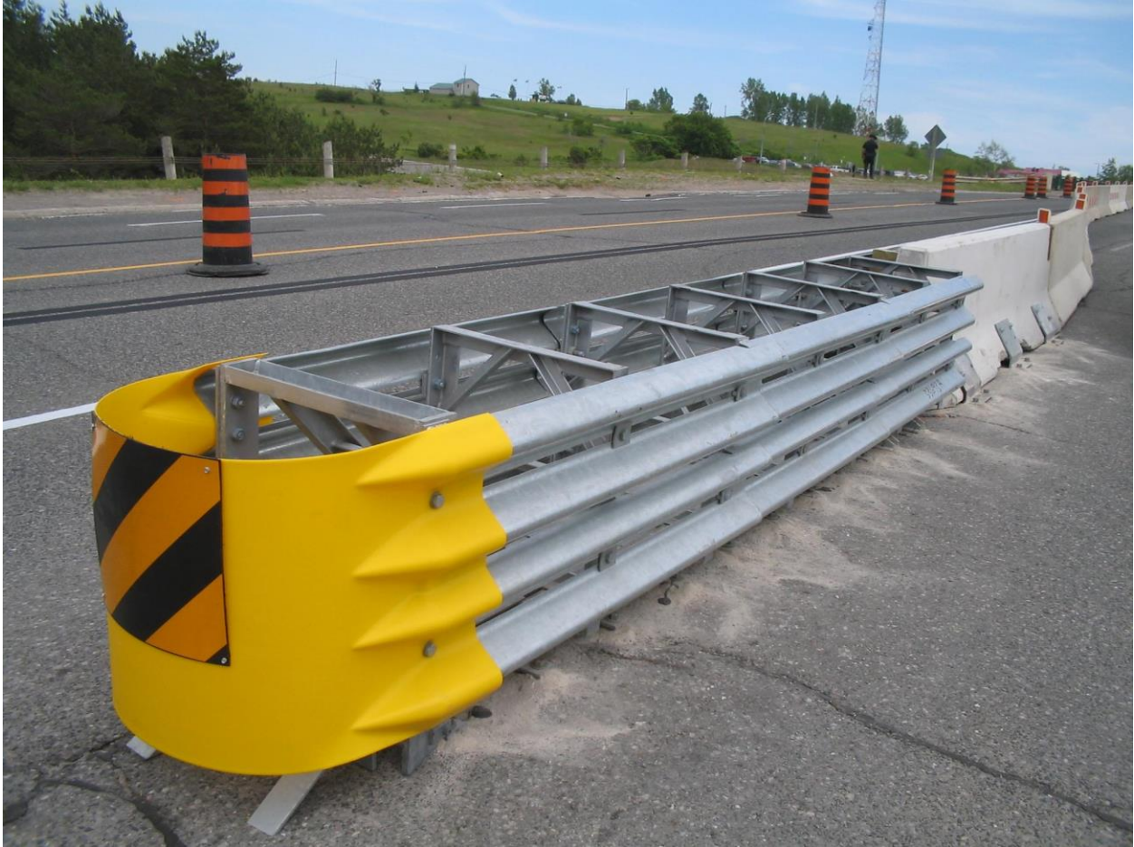
Figure 3. Typical TRACC System
